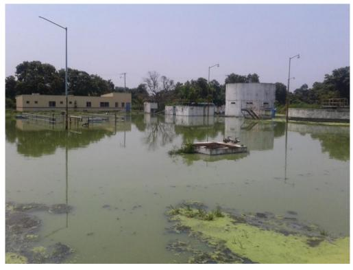
**Figure 1.** Abandoned wastewater treatment plant in the municipality of Ciuhuatlán, Jalisco. The wastewaters are still collected in an extemporary pond flooding the WWTP.
