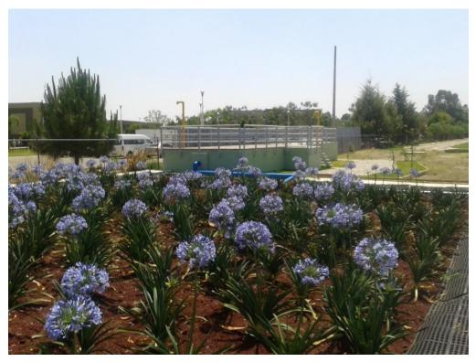
**Figure 4.** Treatment system located in Zapopan, Jalisco, based on a septic tank, anaerobic filter and artificial wetland which operates according to local water quality standards (Courtesy of CIATEJ).
