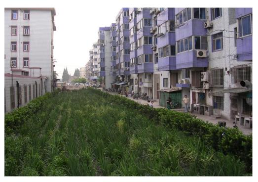
**Figure 5.** Wastewater treatment system based on anaerobic processes and artificial wetlands in Huaxin, Shanghai, China (Courtesy of Janisch & Schultz).
